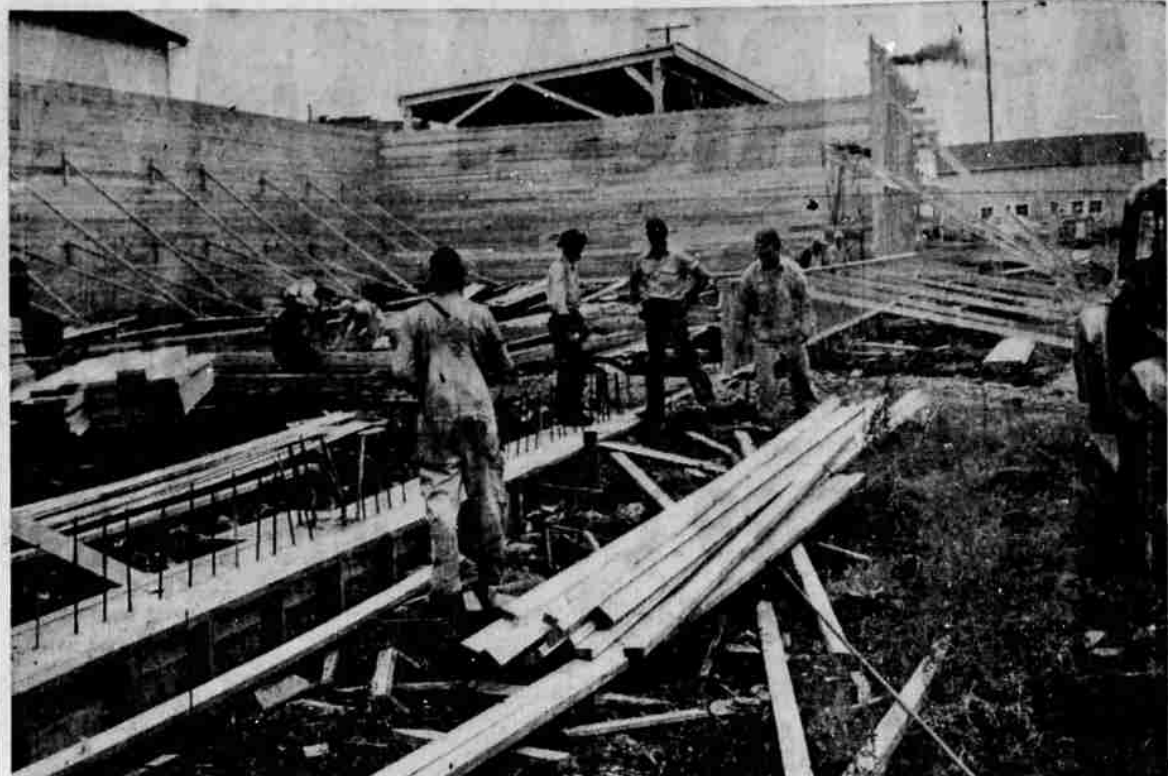
CONSTRUCTION UNDERWAY —California Oregon Power company's new warehouse rises on the company's lot on East Second Avenue So. Permit was issued earlier in July for $47,000. This building is the second in the company's plans to erect four structures for its expanded needs in the Roseburg area. (Picture by Paul Jenkins)
