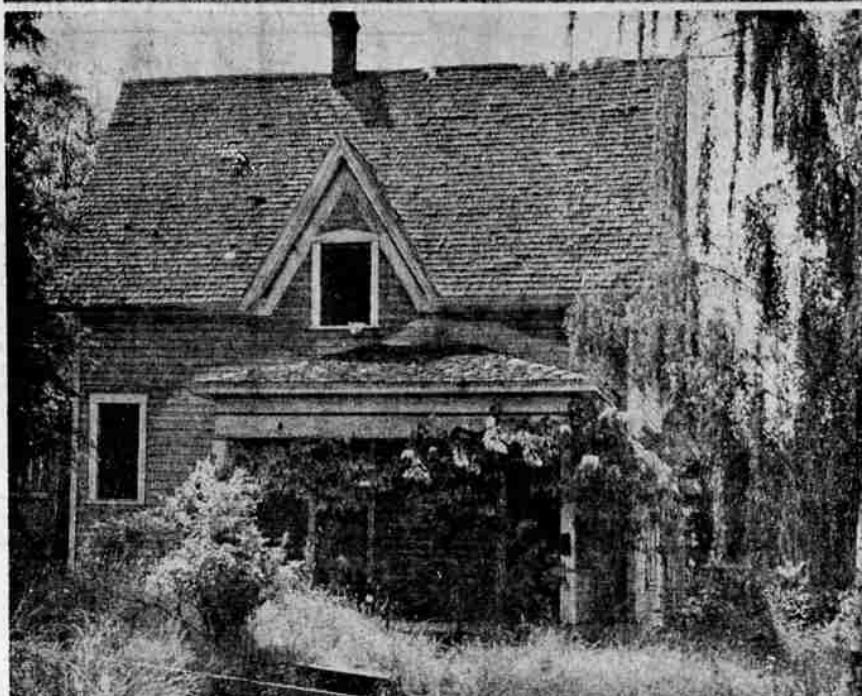
DEMOLITION — Two homes, which have served their purpose in Roseburg, are in the process of being torn down, according to City Inspector C. H. Boniols. The home in the upper picture is located at 220 So. Rose street, and is owned by Orville Munson. It is being demolished voluntarily by its owner. The lower picture shows the home, located at 352 South Main street and owned by William A. Oerding. The building was condemned by the city, said Boniols. (Pictures by Paul Jenkins.)
