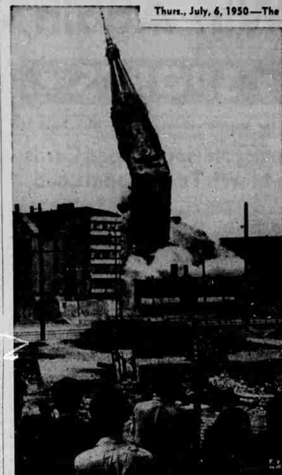
CHURCH STEEPLE BLOWN UP—The steeple of St. George's Protestant Church is blown up by an East Berlin demolition squad after Communists declared it a safety hazard.
