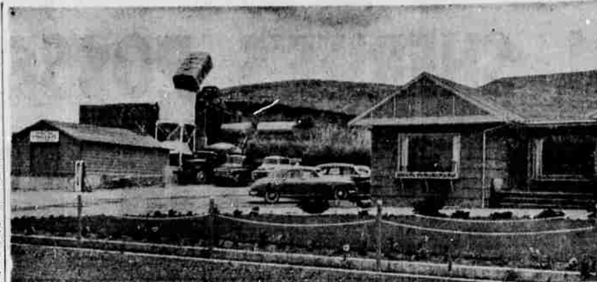
ESTABLISHED TWO YEARS—The I-Deal Concrete Co., owned by Mr. and Mrs. Frank Rogers, has been established two years. The plant has six full time employees, operates six trucks, including mobile mixers, bunkers and a tractor. The daily capacity is 125 to 150 yards of mixed concrete. Approximately $100,000 has been invested in the home, plant and equipment. The company has poured such jobs as Mercy Hospital, county home, Riverside school, REA building, Pine Motor Theater, Benette theater and many homes and private construction jobs. (Picture by Paul Jenkins).
