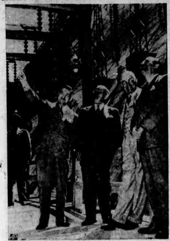
TRUMAN AT COULEE DAM —President Truman inspects the transformer deck of Coulee Dam at Grand Coulee, Wash., prior to the dedication of the largest concrete structure on earth. Left to right: A. F. Darland, supervising engineer; Truman; Frank A. Banks, district manager of the Columbia Basin Project, and Senator Magnuson (D-Wash.). (AP Wirephoto).
