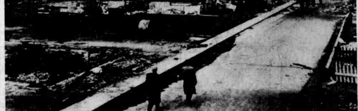
FIRE-GUTTED BUILDINGS AT RIMOUSKI, QUEBEC —The center of town of Rimouski, Quebec, is nothing but ruins after being gutted by a $20,000,000 fire. More than 2,000 were homeless after being burned out by a fire that started at one of the town's lumber yards. A third of the town is a smoldering ruin.
