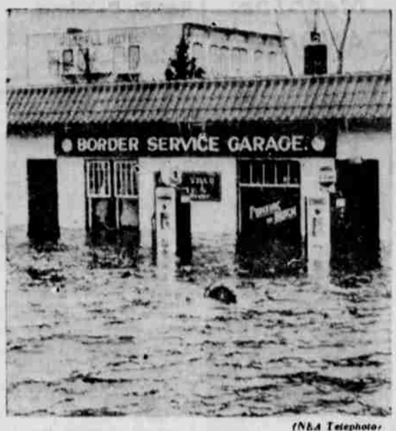
BORDER SERVICE GARAGE. (N.A. Telephone) HARBORIZED—This service garage in Emerson, Manitoba, Canada, is flooded, but not with business. Waist-deep water surrounding the station is part of the flood which has plagued Southern Manitoba and Northern Minnesota for more than a week. It's hardly the place for cars, but motorboats couldn't ask for a better port.
