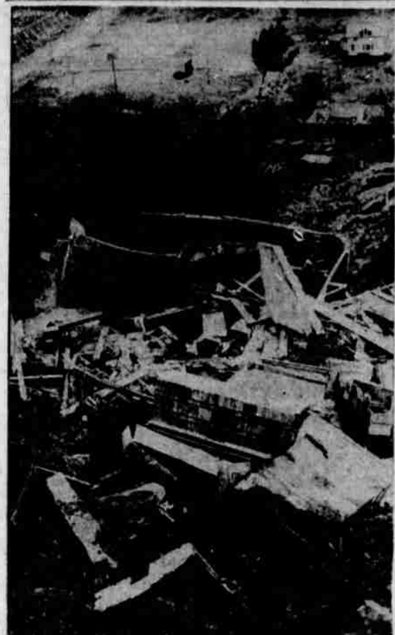
DEMOLISHED BY CREEPING HILL —House lies in shambles on creeping Cooxcomb hill in Astoria, Oregon, where in three months a slithering earth flow has demolished or damaged 21 homes. On the north side of the same hill, geologists warn of a potential slide forming that would do much more damage than the present landslide. About 50 per cent of the city's 18,000 residents live on the north slope. Cooxcomb hill damage is estimated at $150,000 (NEA Telephoto)
