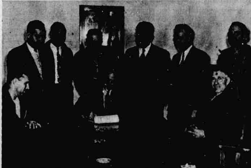
HOSPITAL CONTRACT SIGNED—John Todd of Todd Building Company, seated center, Tuesday signed the $392,900 contract for construction of the new Douglas Community hospital. Immediate action on the contract was taken by the hospital directors after they had earlier in the day received word that the hospital plans and additional federal funds had been approved by the U. S. Health Service in San Francisco. In the picture, left to right, are Dick Gilman, hospital Director A. Knauss, Gordon Todd, Harold Hickerson, Dr. Roy Hanford, Daniel R. Dimmick, Buckley Bell and Frank Ashley (seated). (Picture by Paul Jenkins).
