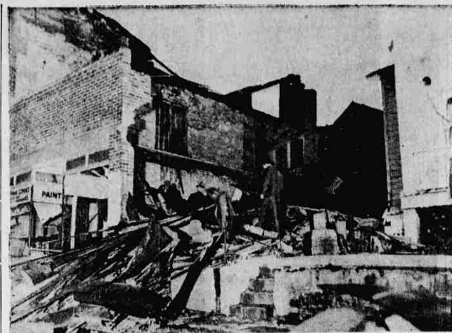
TORNADO TOLL HEAVY —Men dig through the rubble of a building in Hannibal, Mo., looking for their belongings after a tornado struck the community. No one was killed, but 11 persons were injured. Property damage in Arkansas, Oklahoma, Illinois and Missouri was high, with Arkansas alone estimating more than $100,000 damage caused by the twister.
