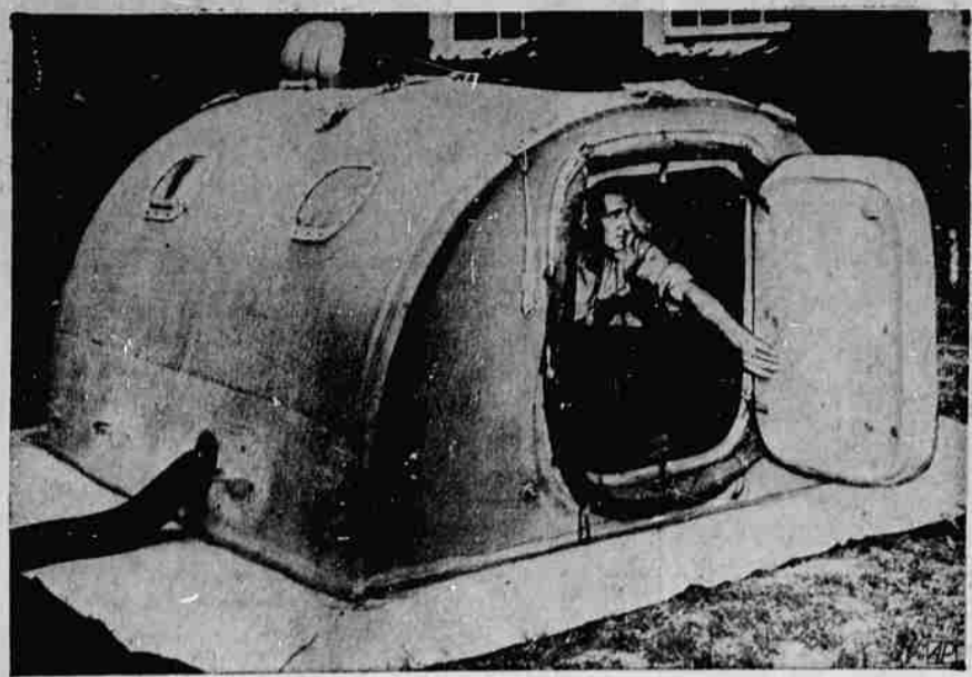
BLOWUP 'QUONSET' HUT—This pneumatic Quonset hut, developed for use in Arctic areas, can be inflated with a simple hand pump in three minutes. The Defense department, which released this photograph, says the hut is snow, water and draft proof and has air-light plexiglass windows; it can support about 500 pounds and can withstand winds of 100 miles an hour. The hose at left is an air duct for ventilation.—AP Wirephoto.
