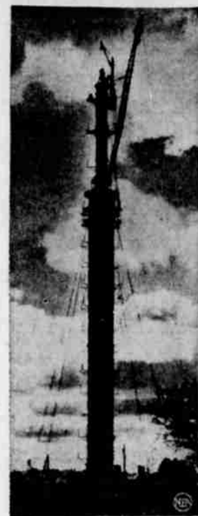
ROCKET LAUNCHER? —Motorists on the outskirts of Dallas, Tex., kept expecting this tall, rocket-shaped thing to take off. Having seen pictures of the rocket launchings at White Sands, N. M., they called the papers to find out when this one would be launched. The papers investigated and found the "rocket" was one of the legs for a huge water tower being built at a housing development.
