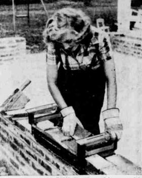
BRICKLAYING MADE EASY—The "first real improvement in five centuries in the method of laying bricks" is demonstrated in Montgomery, Ala., by coed Kitty McGlynn. The device, invented by engineers Paul H. Sommers and John S. Hodgson, is said to speed bricklaying four times the normal pace. Acceptance by the building industry could mean great savings in construction costs—especially in the building of low-cost homes.
