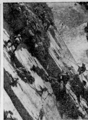
ALPINE CLIMBERS? NOPE-Except for their hard hats and world's fourth largest concrete dam, across the Flathcad River. These jacknammermen are drilling holes to prepare for blasting the caryon wall down to the solid bedrock that will support the dam. So steep is the wall that two men are required on each jacknammer.
