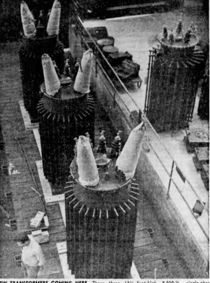
NEW TRANSFORMERS COMING HERE-These three 121/2-foot-high, 8,000-lb., single-phase transformers were made at the General Electric company's transformer manufacturing plant located in Oakland, Calif. Rated at 500kva, 66,000 volts each, they are destined for the California-Oregon Power company's Carnes substation, south of Roseburg. There they will add power needed for a fast-growing agricultural and lumber area.
