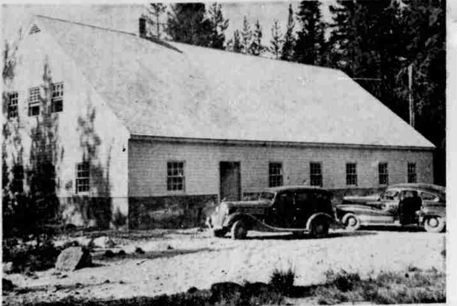
NEW HATCHERY AT DIAMOND LAKE —Finishing touches are being applied to the new Diamond lake hatchery building pictured above. Located on Lake creek, outlet to Diamond lake, the new building replaces an old structure so weakened that it had to be propped with poles. The new hatchery greatly increases capacity for handling rainbow trout eggs taken from the lake. Improvements also are contemplated at the nearby residences and other structures connected with the egg-taking station.
