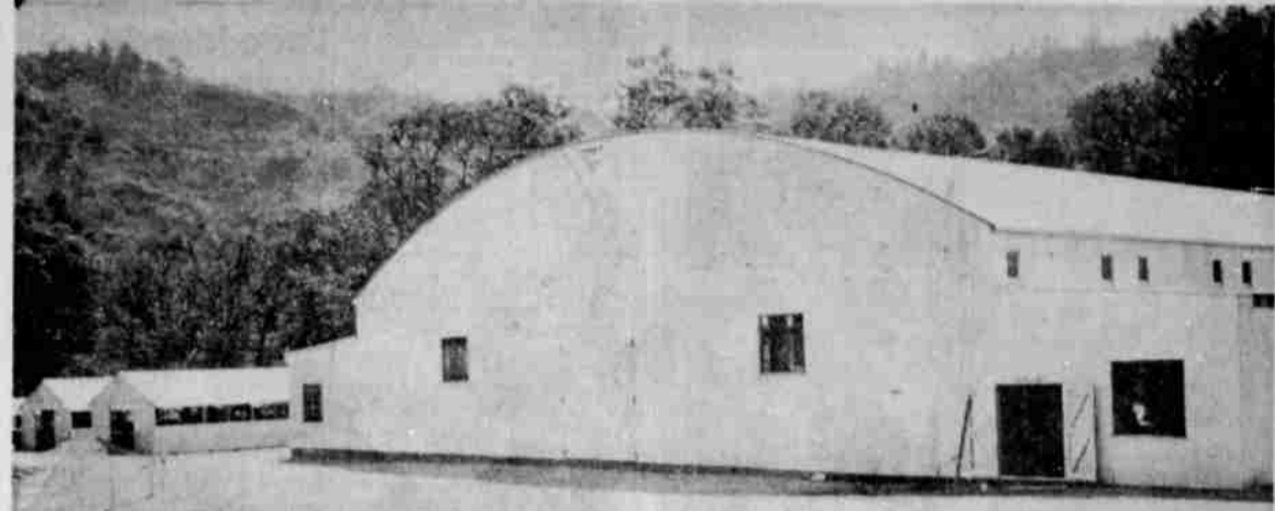
NEW FAIR BUILDINGS —This new 100x140 exhibit building has been erected for the first Douglas county fair in 37 years. On its exhibit floor will be arranged community booths entered by organizations throughout the county, large farm equipment displays, commercial exhibits, and 4-H club entries. In the background are the two livestock barns to be used by the 4-H and Future Farmers of America. The fair will open tomorrow for three days. (Picture by Photo Lab)
