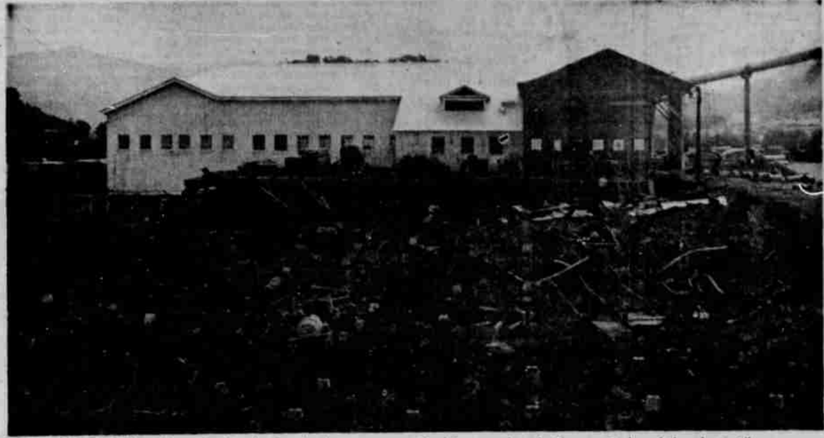
PLANT LOSS HEAVY —Above is the Trojan Lumber company manufacturing plant at Riddle, after it suffered a $100,000 loss Aug. 6. Cause of the fire was undetermined. Destroyed were the edger, trim-saw, green chain, re-saw and the dock. The planing mill and sorting platform were saved. According to D. W. Gill, the planer is expected to resume operations the first of the week, after supporting timbers, partially burned,
