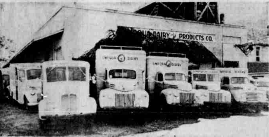
PROOF OF EXPANSION is shown in this photo taken 14 years later. Not only had the two partners expanded their truck fleet from one to nine, but they also occupied a much larger, especially designed building. This building is the present site of the Umpqua Dairy, located on the corner of Sykes and Short streets.
