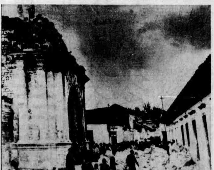
IN ECUADOR QUAKE—Shown above is the tower of LaMerced church in Letacunga, summer resort of Quito, as it crumbled during the Ecuadorian earthquake this week. At least 50 towns were demolished, approximately 6,000 persons killed, 150,000 others made homeless, and property damage of at least $20 million inflicted.
