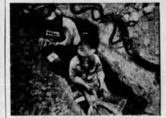
1. When someone's ditch-digger bites a chunk out of a long distance cable - and it happens now and then - repairmen get on the job fast to fix it. Back at a test center, sensitive instruments located the break and splicers hit the road. Almost simultaneously, many calls were routed through other cities to get them. through with as little delay as possible
