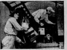
2. Service restored ... the hundreds of tiny wires have been spliced temporarily and, even as the workmen stow their tools, calls are speeding through the cable. Later it will be per-manently spliced without interrupting service. Such fast repairs are possible by planning ahead for emergencies, so trained people can be quickly pulled from other jobs.
