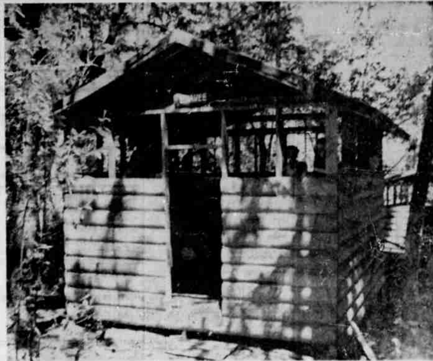
LIVING UNIT —One of the Camp Fire Girls' cabins at Camp Tye is pictured here. Ten of these cabins have been built at the camp to provide comfortable shelters for the girls. All construction has been done by volunteer labor from Roseburg and Drain civic groups and fathers of participating girls. (Picture by Paul Jenkins)
