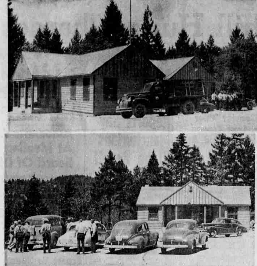
GAZLEY STATION —Pictured above are views of the south Douglas branch of the Douglas Forest Protective association, inspected by directors, timbermen and foresters Wednesday. Located at Gazley, north of Canyonville, this new station was completed for use early this summer. It has a complement of 20 men under the supervision of Bruce Ferguson. The upper picture shows the headquarters building used as sleeping quarters and dining hall, with the cook's quarters in the rear. The lower picture shows the equipment building. (Pictures by Paul Jenkins)
