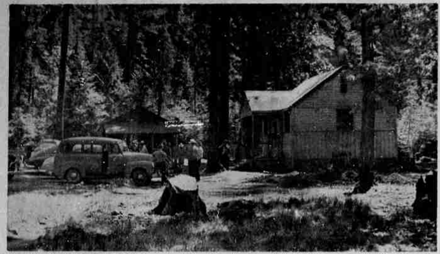
SOUTH MYRTLE CAMP —This branch of the Douglas Forest Protective association's fire patrol located on South Myrtle creek is scheduled to be discontinued, now that the large station has been constructed at Gazley. The facilities would be moved to the Glendale-Azalea area as soon as access roads are put in. The station was visited by directors and foresters on an inspection tour Wednesday. (Picture by Paul Jenkins.)
