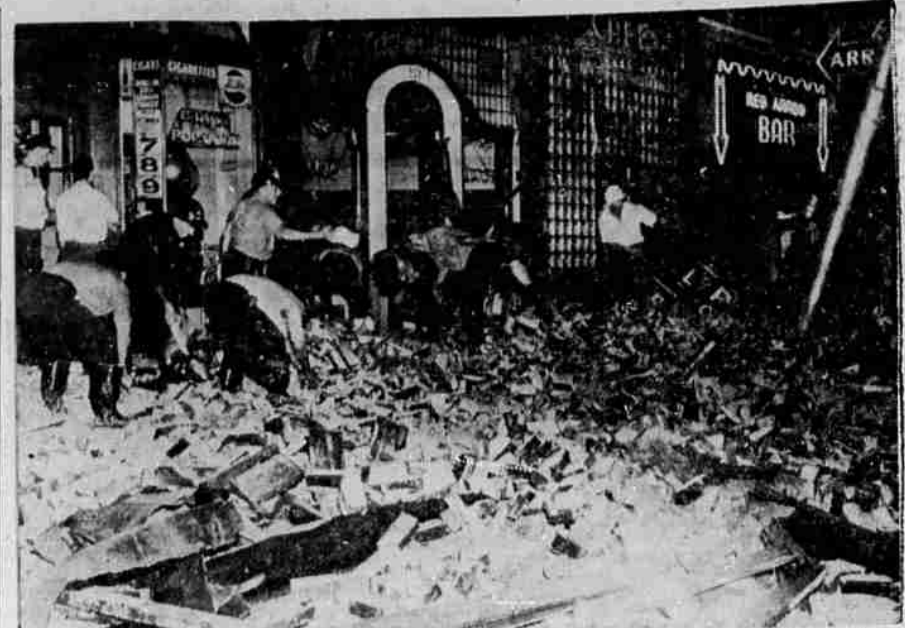
BUILDING FRONT COLLAPSE KILLS FOUR —Firemen and rescue workers clear the rubble of bricks that crashed to the street in Pittsburgh, Pa., killing four persons and injuring eight, four critically. A large neon sign weakened and collapsed the brick parapet atop the one-story building, showering the bricks onto the street below.
