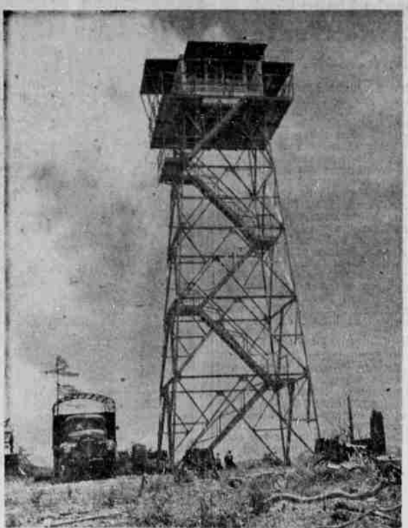
NEW LOOKOUT TOWER —Forty-four-foot steel tower has been erected on Mt. Chivigny, on the Little River-North Umpqua divide. It was constructed under supervision of the Douglas Forest Protective Association and will be manned by Forest Service lookouts this summer. (Forest Service Photo.)
