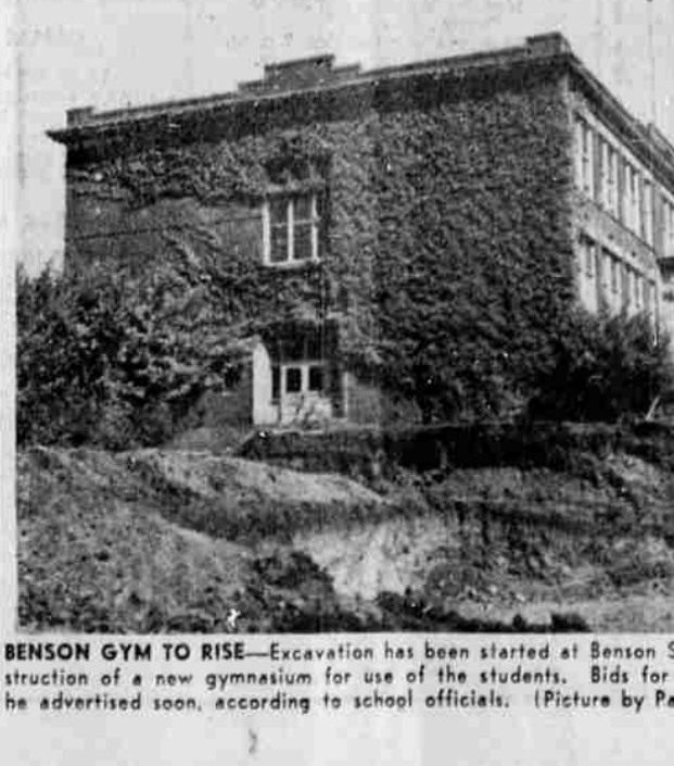
BENSON GYM TO RISE—Excavation has been started at Benson School preliminary to the construction of a new gymnasium for use of the students. Bids for erection of the structure will be advertised soon, according to school officials. (Picture by Paul Jenkins).
