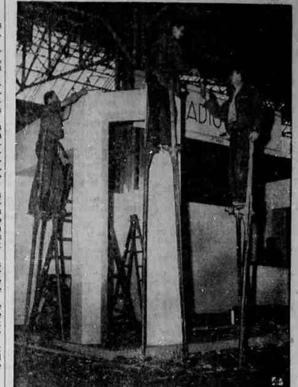
CARPENTERS ON STILTS —Stilts replace ladders for carpenters building stands for the Fair. Workmen say they move around better and the stilts cost less than ladders.
