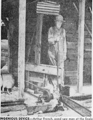
INGENIOUS DEVICE—Arthur French, pond saw man at the Engle and Worth mill near Canyonville, operates the controls of a saw equipped with an ingenious device—a water-jet apparatus which washes away the sawdust after logs are cut. The water jet is not operating in this picture. This pond saw is soon to be moved to the opposite side of the pond from its present location. (Picture by Paul Jenkins.)
