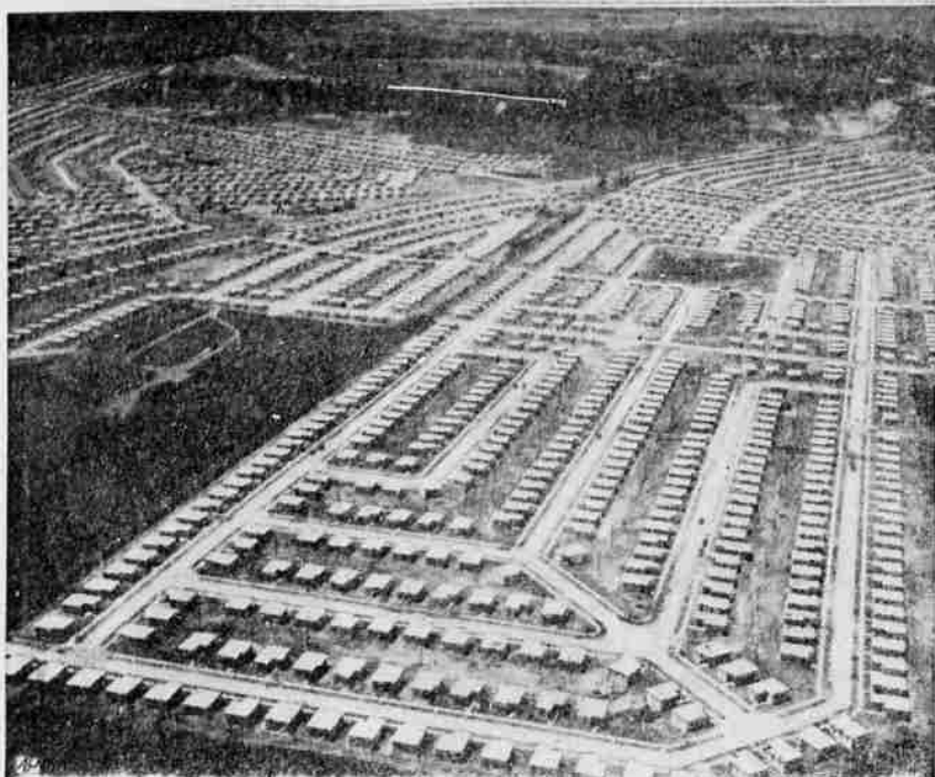
HOUSES BY THE THOUSAND —One of the world's largest private housing projects is near San Juan, Puerto Rico, where 3,500 homes are occupied and 1,500 more are under way.
