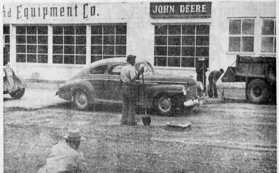
GETTING READY TO PAVE —Traffic here moves slowly over E. 2nd Ave. S. as workers spread gravel from a truck. In a preliminary step to street paving. As part of the North Umpqua Highway, E. 2nd Ave. S. will be paved with asphaltic concrete from N. Jackson St. to the east city limits. Work is expected to get underway this summer. (Picture by Paul Jenkins.)
