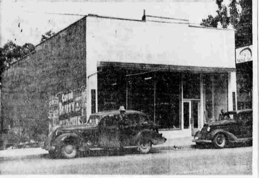
OCCUPIES OLD SITE—This Firestone store, owned by I. N. and Ralph Gray, stands on the site of the old Masonic building in Canyonville, which burned a year or so ago. It is across the street from another store owned by the firm, where the old Canyonville Hotel formerly was located. This unit houses the hardware and appliance departments and is managed by the owners. (Picture by Paul Jenkins.)
