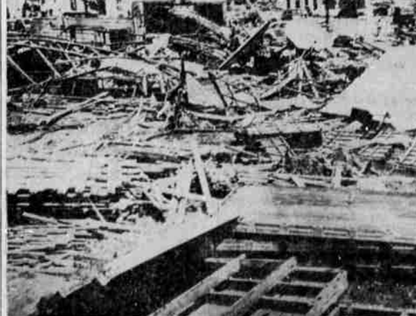
FLATTENED BY TORNADO —Five persons were killed and 83 others injured when a tornado Sunday night struck Amarillo, Texas, with the result pictured above. An estimated 350 homes in a 35-block area were either demolished or mangled. The tornado was the first of a series of storms that struck portions of Texas and Oklahoma, leaving 14 dead, 138 injured, thousands homeless, and inflicting several million dollars damage.
