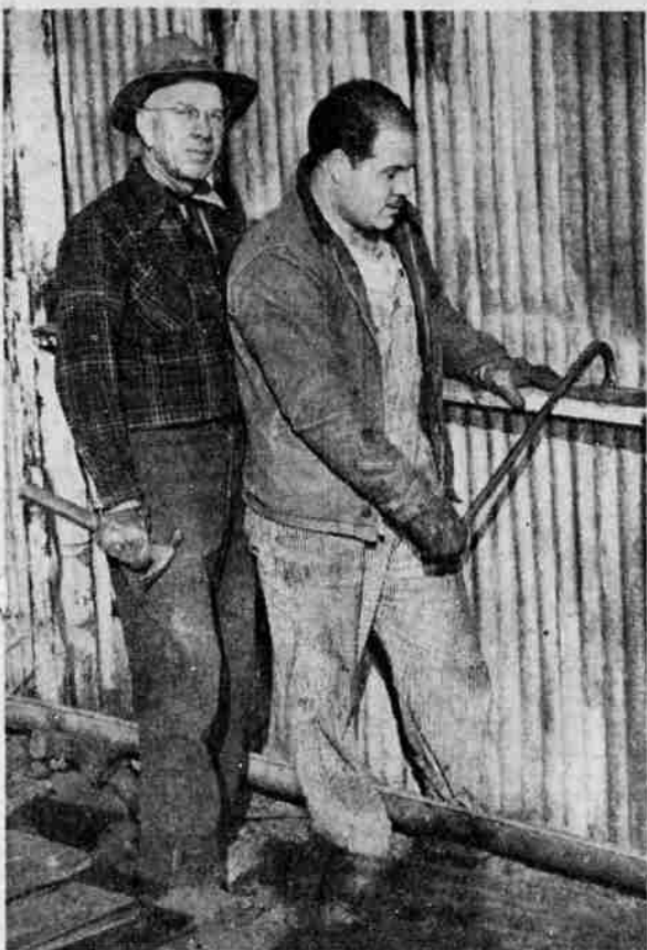
W. J. (BILL) ADAIR, at the left in the picture above, and JACK ADAIR, his son, are tearing down the last section of the old lumber yard buildings which through endless years have occupied but not adorned the half-block lot at the northeast corner of Main and Washington Streets.
