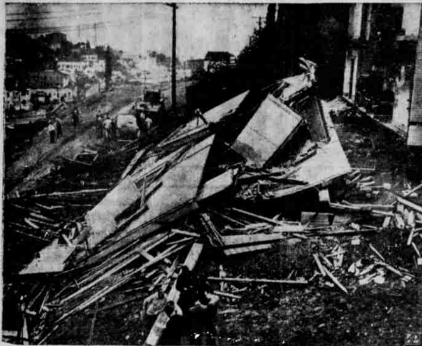
HOUSE MOVERS ESCAPE DEATH IN COLLAPSE —Six house movers, eating their lunches under this newly-moved apartment house in Los Angeles, miraculously escaped death when the two-story frame building collapsed. The front section of the building had just been lowered to its new foundations when it crumpled and splattered into a pile of rubble. Six scared movers crawled out from underneath—none of them even scratched. (AP Wirephoto)
