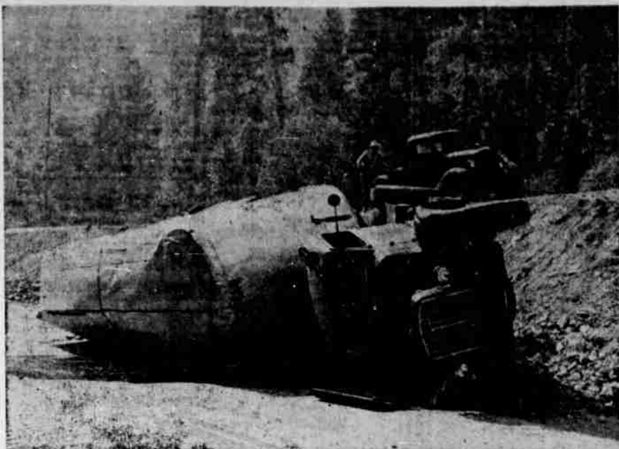
TRUCKS PREFER OLD HIGHWAY —Scores of persons who attended the dedication of rebuilt portions of the Pacific Highway near Wolf Creek were intrigued by the sight of a large, fully-laden produce truck lying on its side two miles north of Wolf Creek. This picture was taken by Robert Martin of Grants Pass before the wrecker arrived. The unidentified driver is said to have told passersby that his brakes locked and he lost control. In any event, the truck flopped off the new highway onto the old route, which it formerly traveled, alongside.
