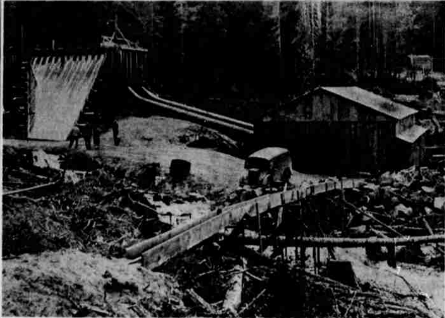
GENERATING PLANT SERVES TOKETEETEE PROJECT —Pictured above is a newly installed hydroelectric plant, located on Clearwater river, providing power for the Copco camp at Toketeetee Falls and the tunnel construction job at Slide Creek. John C. Boyle, vice-president and general manager of The California Oregon Power Company, installed the unit, which uses water carried by viaduct from Clearwater, and dropped through two penstocks to turbines, driving 2300-volt generators. A spillway carries off surplus water from the reservoir. The hydroelectric plant replaces diesel power plants formerly used. The plant will be removed when the Toketeetee power station is complete, as the ground area will be flooded by water from the 75-foot diversion dam.
