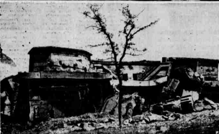
NAZI BUNKER BLASTED —The Zoo Bunker, wartime air raid shelter in Berlin, is blasted by a charge set off by British engineers. Top: The explosion. Bottom: The remains.
