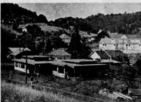
ANIMAL HOSPITAL —Dr. Dallen H. Jones, veterinarian, is building the Roseburg Animal Hospital on North Stephens Street.
