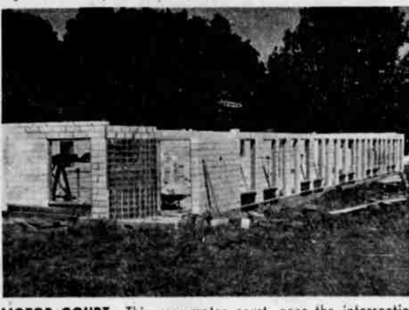
MOTOR COURT —This new motor court, near the intersection of Winchester Street with North Stephens Street, is being built by Chet Hamm.
