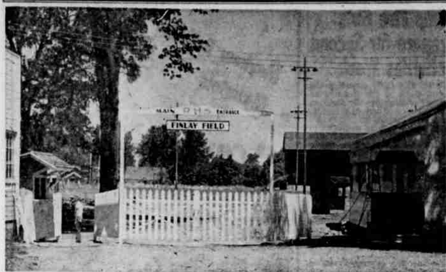
NEW FIELD ENTRANCE —A new gate and ticket booth have been added to Roseburg's Finlay Field as part of the rejuvenation program underway. The new industrial arts building, left, and the new band room, right, are also included in the school additions, under the direction of Building Supervisor J. W. Mess. Future plans call for a mud-free path to the football stadium, more bleacher seats, and a running track which is now under construction.
