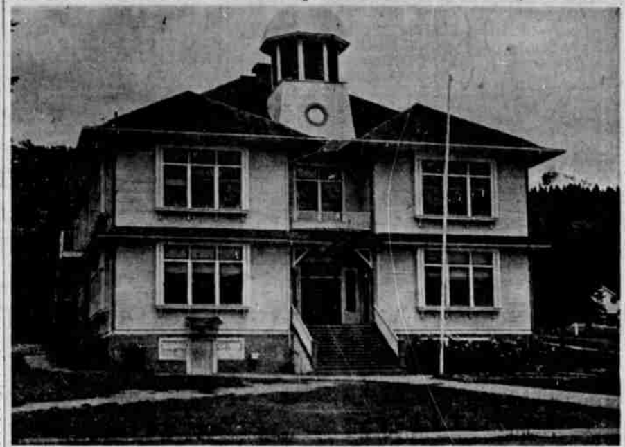
SUTHERLIN SCHOOL CONDEMNED —The 37-year-old Sutherlin High School building pictured here has been condemned for use as a school building by the State Department of Education and will be replaced by a new building to be started this summer, said Superintendent of Schools William W. Riddlebarger. This old building will probably be razed.
