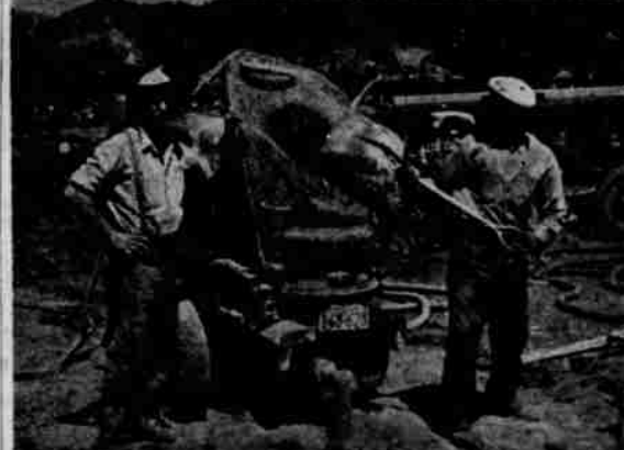
NEW RESERVOIR FOR DRAIN —Above is seen the new 650,000-gallon water reservoir nearing completion at Drain. Concrete is blown on the sloping sides and bottom of the tank by means of compressed air, as seen at left. The dry cement and crushed gravel is shoveled into the machine which blows the mixture through a hose. Water is added at the nozzle. The concrete mixture is tamped under 45 pounds of air pressure.
