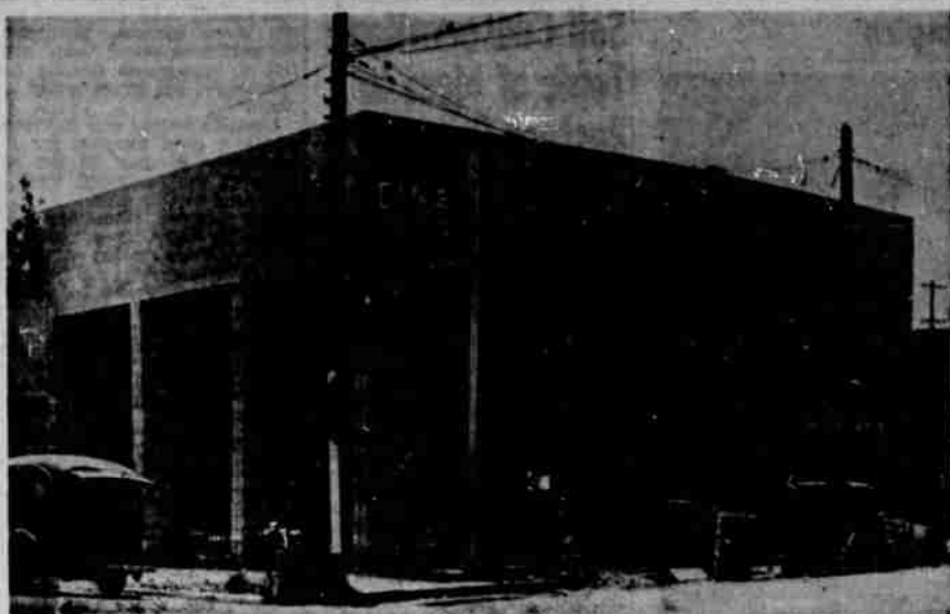
NEW BANK BUILDING RISES —The United States National Bank's Douglas County branch, now at Yoncalla, will occupy this new building in Drain. The move is expected to be made sometime during August, said J. H. Innes, manager. The building is 35 x 48 feet, constructed of pumice blocks. A reinforced concrete vault at the rear will contain 500 safe deposit boxes. There will be a mezzanine floor on top of the vault. C. A. Catching of Drain is contractor for the $35,000 project. The U. S. National of Portland announced plans to move to Drain when it purchased the Farmers Security Bank of Yoncalla recently.
