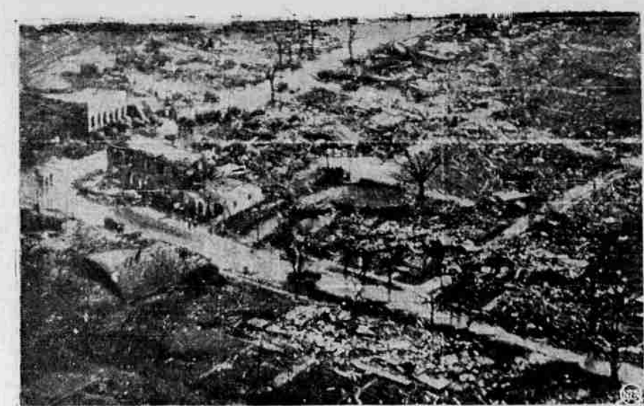
VIOLENT STORM LEVELS INDIANA TOWN —A few badly damaged brick and stone buildings are all that remain of the business district of the small town of Coatesville, Ind., after a tornado ripped through, killing at least 13 persons. New storms throughout the midwest during the violent 24 hours raised the nation's loss to 56 dead and missing and more than 400 injured.
