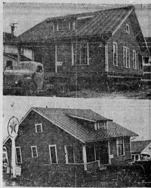
UNCOOPERATIVE RESIDENCE —The sign on the house says "House Moving" but the house was uncooperative. When movers attempted to take the residence at 620 Stephens St. from its foundations, the building slipped off the cribbing and virtually buried the lowboy truck on which it was mounted in black mud, as pictured in the top photo above. By use of trucks, winches, wreckers, etc., enough power was obtained to eventually drag the house and its supporting trailer from the mud and transfer it to a new location at the corner of Thompson and Roberts streets. A commercial building will rise on the Stephens street site.
