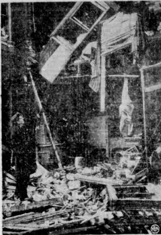
(NEA Telephoto) Three persons were injured in a gas explosion which wrecked this Pittsburgh, Pa., apartment house, causing damage estimated at $2500. One victim was pinned under the debris for a half hour before firemen rescued him.
