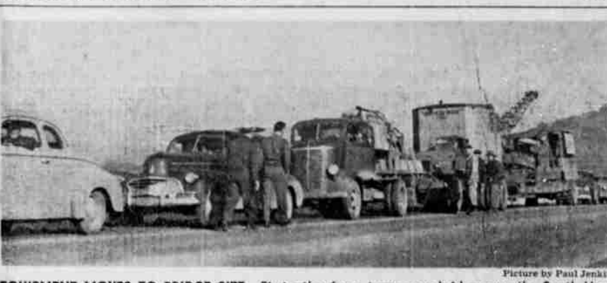
EQUIPMENT MOVES TO BRIDGE SITE—First piles for a temporary bridge over the South Umpqua River near Dillard were driven last night by Ben Doerksen, Roseburg contractor. Bridge building equipment is pictured above, as it moved to the bridge site Friday.
