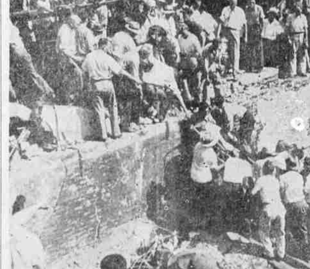
BLAST RIPS BEAUTY SHOP, KILLING TEN —Police and volunteer workers remove an injured victim from the basement of a Harrisonburg, Va., beauty shop and school which was completely demolished by a coal dust explosion. Ten women were killed and about 30 injured. Blast blew out the back wall of the building and so wrecked the front wall that a crane had to be used to remove the hazard.
