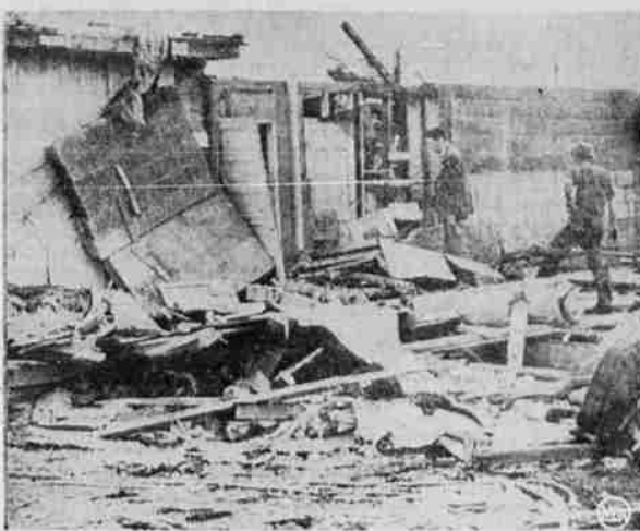
Scattered over a three-block area was this home in residential section of Champaign, Ill., which was struck by a tornado. The family took shelter in the basement. No fatalities were reported, although six homes were completely demolished and 25 others were damaged.
