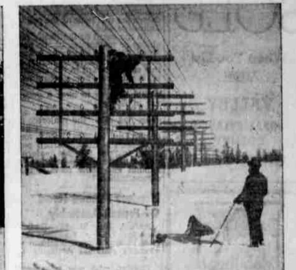
Enough men rush to the job to keep repair work going without stop . . . in the meantime, calls are immediately rerouted whenever possible. And sooner than you might imagine, the damaged lines are in use again. For here, as in everything we're now doing to grow with the West, telephone people work with a splendid spirit of service and teamwork . . . and always with you in mind.
